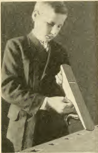
Fig. 12. Setting a Plane.
